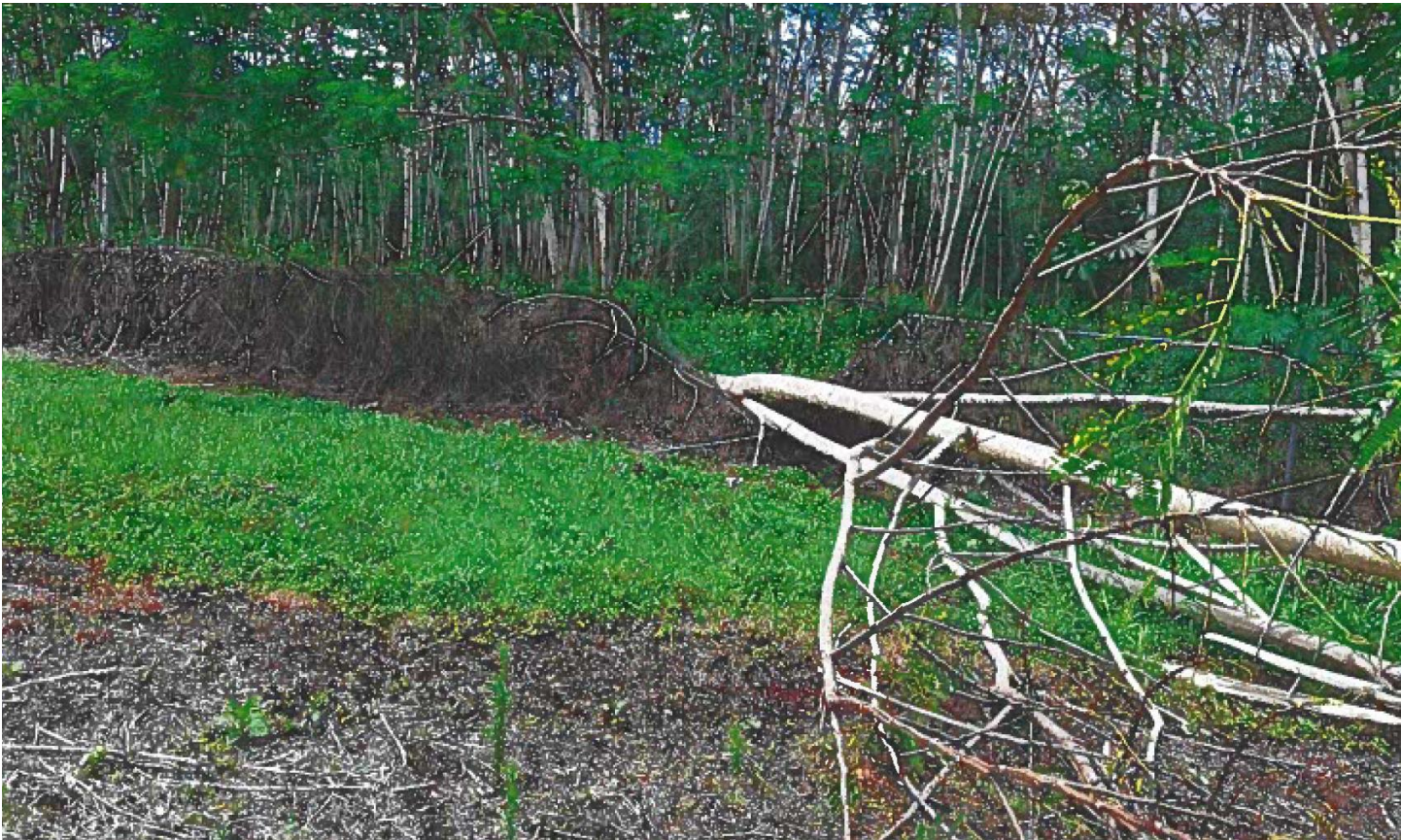
Tree fall over fence
